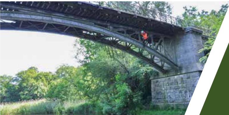
Bridge inspection on Fodsporet performed for The Danish Nature Agency
