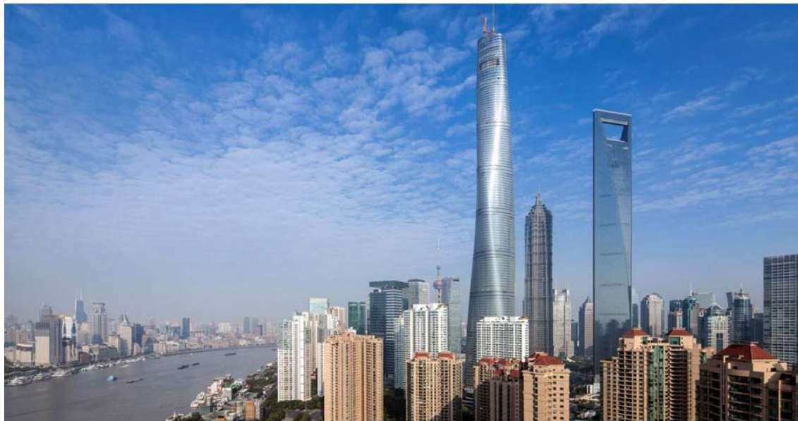
Shanghai Tower, China
