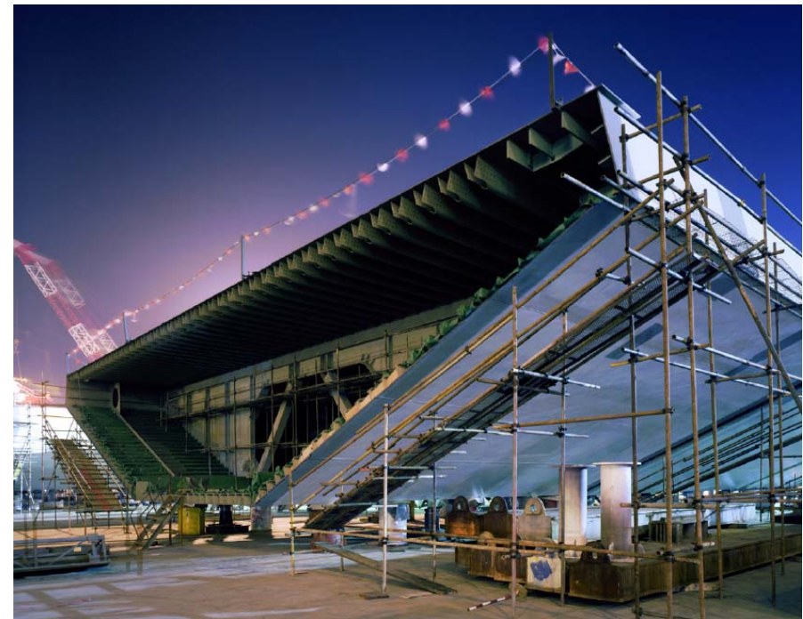
San Francisco Oakland Bay Bridge
